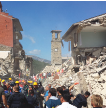
August 24, 2016: Corso Umberto in the historic centre in Amatrice, Italy, reduced to a pile of rubble.
